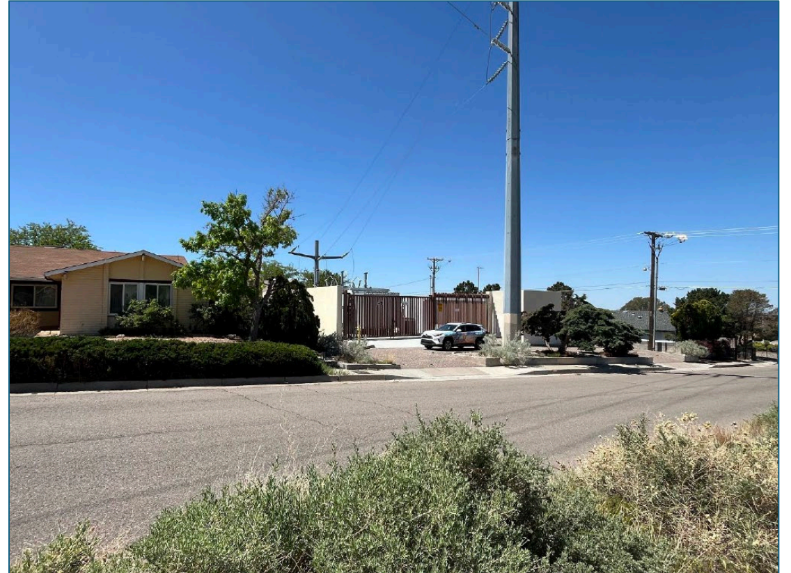
Substation near Crestview Park
