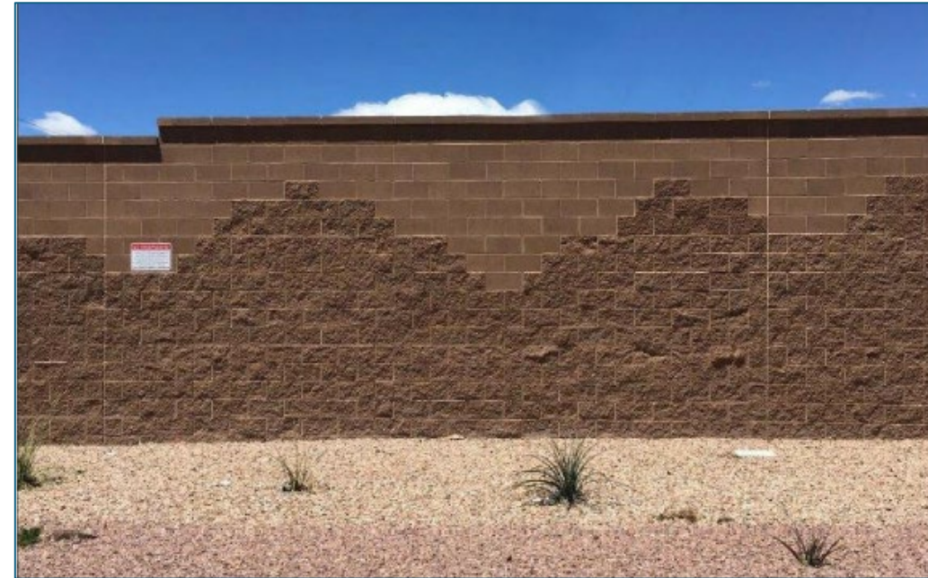
Typical Substation Wall
